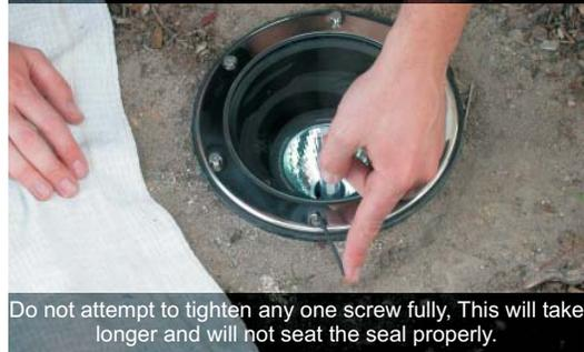
Do not attempt to tighten any one screw fully, This will take longer and will not seat the seal properly.
