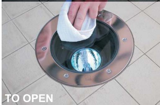
2. Clean out socket head screws with a small pointed object
