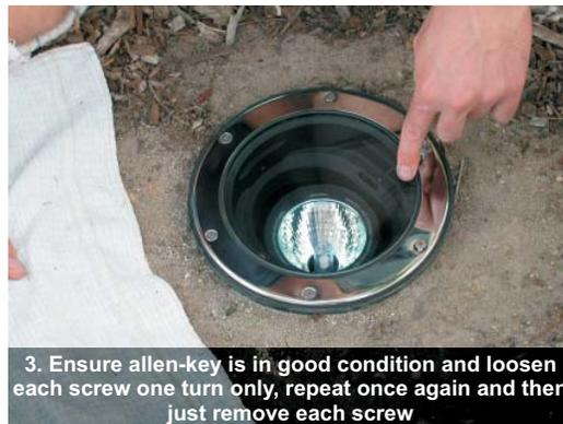
3. Ensure allen-key is in good condition and loosen each screw one turn only, repeat once again and then just remove each screw
