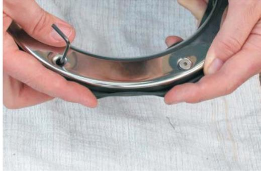
12. Place cover on fixture lining up allen-key with any hole
