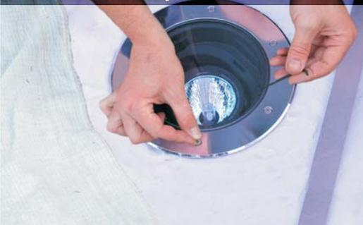
15. Progressively tighten, no torque pattern is required, just keep going around until all screws are tight and the glass, trim and edge of fixture are flush.
